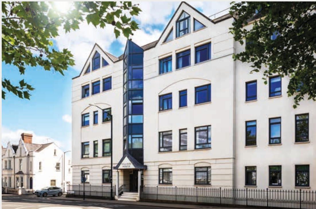
2015 VILLIERS HOUSE, ROYAL LEAMINGTON SPA
